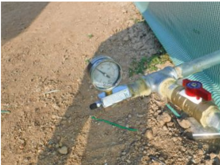
OK- Gas line pressure reading was within acceptable limits.
