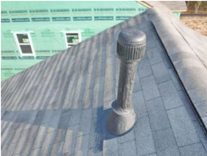
Metal double wall type B vent pipe noted.
