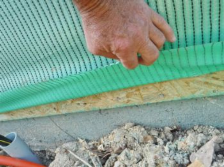
ok- Sheathing and edge blocking appear to be nailed adequately.
