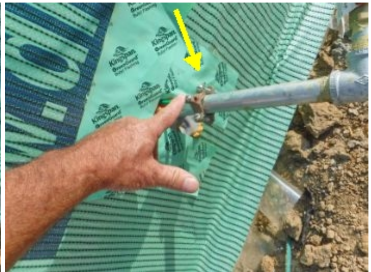
Bonding (loose) - Noted that the bonding clamp was loose at the gas line. It is important that the bonding clamp be tight to the pipe and the grounding conductor. Recommend tighten it up good.
