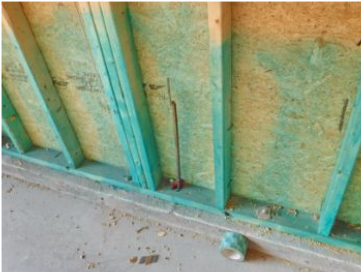
ufer type ground rod shown- incomplete at time of inspection
