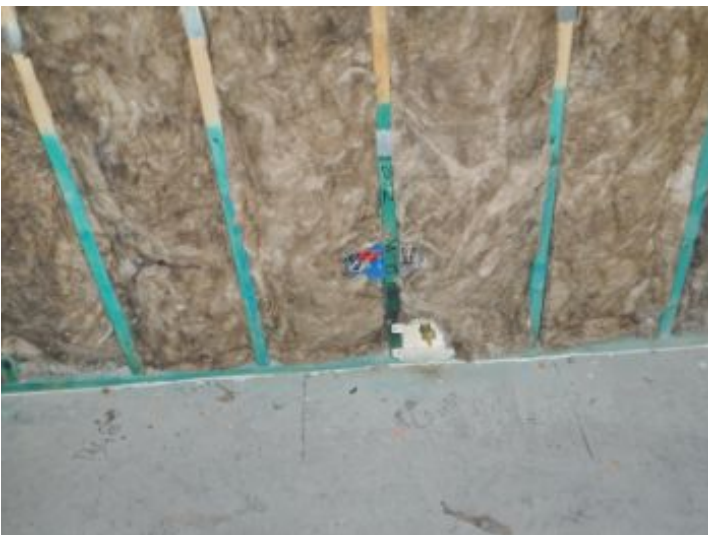
Gas line stub out shown.
