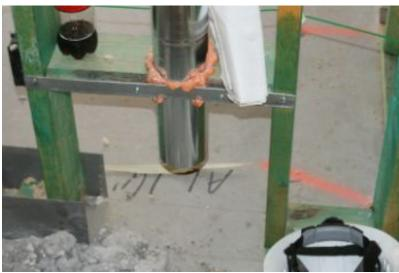
Dryer vent should eventually be fitted with an elbow behind the dryer for proper connection to the metal duct should that area be sheet rocked.
