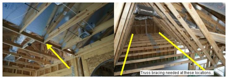
I suggest careful review of the truss documentation which was unavailable for the inspection to see which type of support and connectors are needed here. Typically you would see a girder truss and hangers for the trusses in this area.
