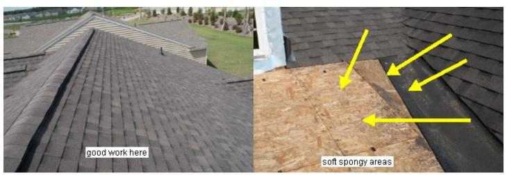
The area in the valley was soft and spongy. I recommend installing support blocks from underneath to reinforce this area.
