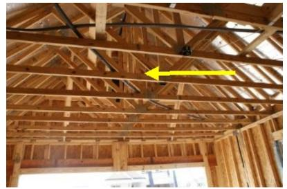
Truss bottom chord was improperly braced. There should be 2x4 lateral bracing on top of the bottom chord of the trusses at less than 10' intervals running perpendicular to the trusses as per standard building practice.
